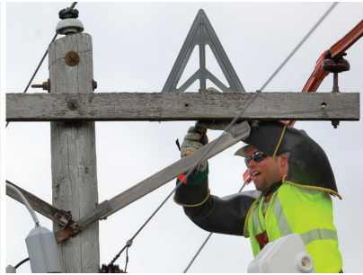
Alliant Energy worker attaches tri- angular pieces of plastic designed to stop large birds from perching along a stretch of power lines where an eagle was electrocuted. Republished with permission © 2015 Iowa SourceMedia Group, Cedar Rapids, Iowa
